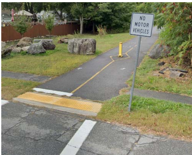
Figure 32 Collapsible bollard in Peabody, MA
