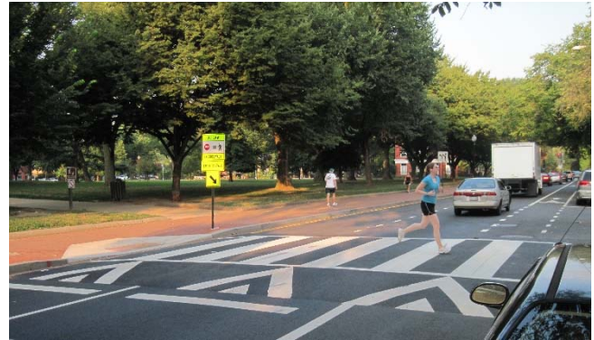
Figure 20 Raised crosswalk in Washington, D.C.
