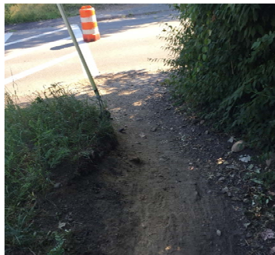
Figure 12 Steep grade entering roadway at Rockaway Ave crossing
