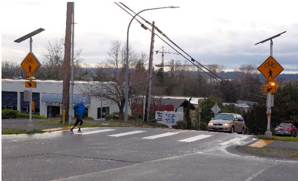
Figure 19 Trail crossing with RRFBs in Kirkland, WA
