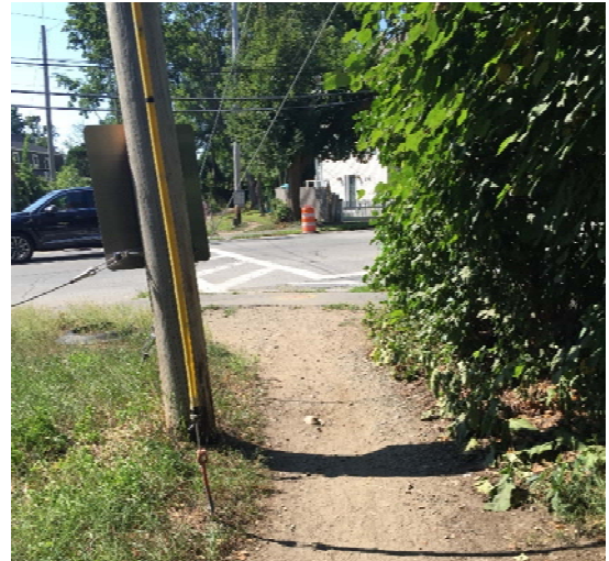
Figure 31 Narrow opening for trail users at Pleasant St crossing with utility wires
