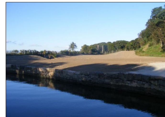
Project site post-remediation and before seeding in 2012.
