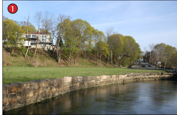
The site can be seen while crossing the “wet” bridge.
