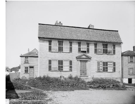
John Glover's House built c.1762
