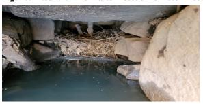
Blockage cleared during storm sewer maintenance
