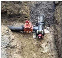
Figure 1 – New Hydrant installed on Crown Way
