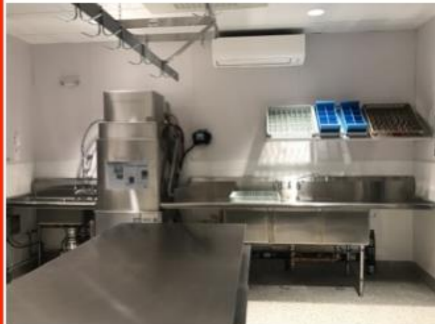
COA Kitchen Renovation
