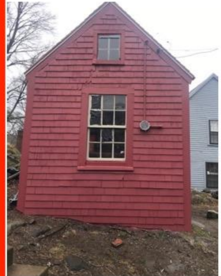
Shoe Shed Renovation
