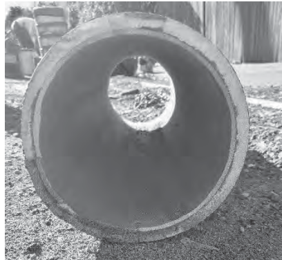
Figure 2 – Interior of the Humphrey Street pipe following cleaning and lining.
