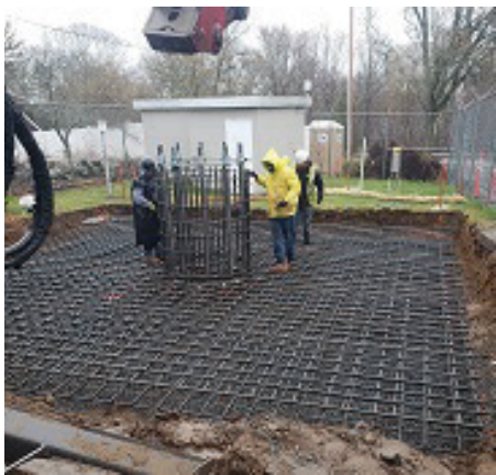
Construction of concrete base
