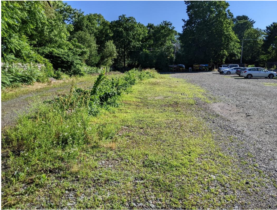
Parking area slopes towards neighboring property along the fence, causing flooding.
