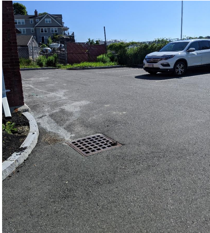
The building's gutter system discharges to the parking lot, causing erosion of the mulch in the garden bed. The bioretention area at the far end also seems to drain to the catch basin, causing discoloration of the pavement.
