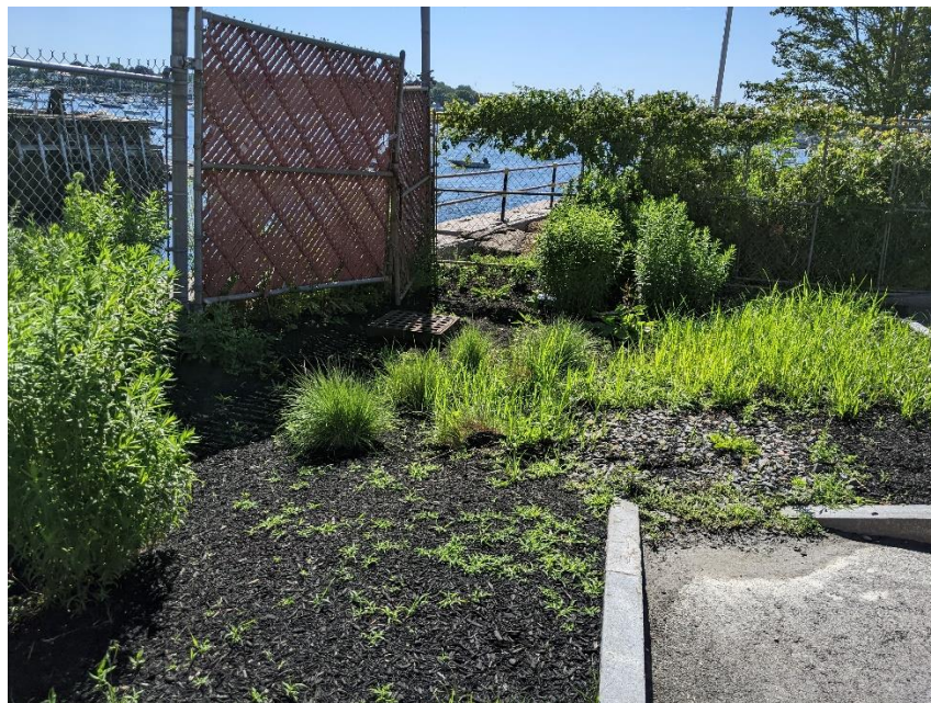
The second bioretention area does not seem to collect and infiltrate runoff effectively. An overflow catch basin also exists in this area.
