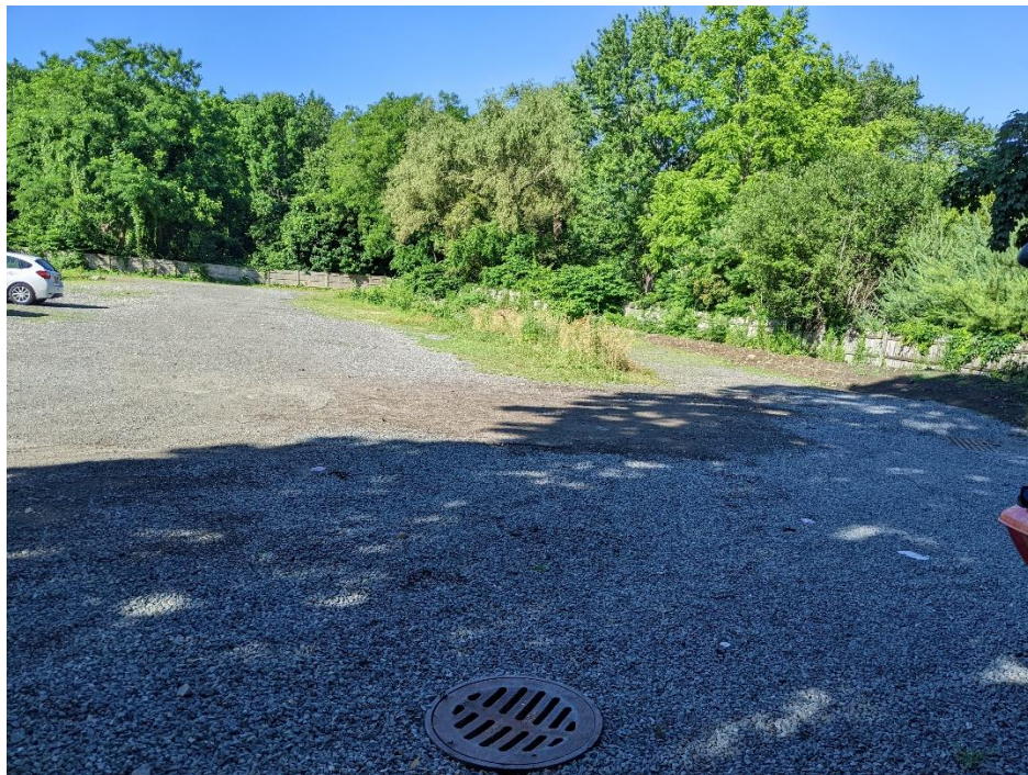
Another catch basin by the entrance of the parking lot. These drain to a nearby priority outfall.
