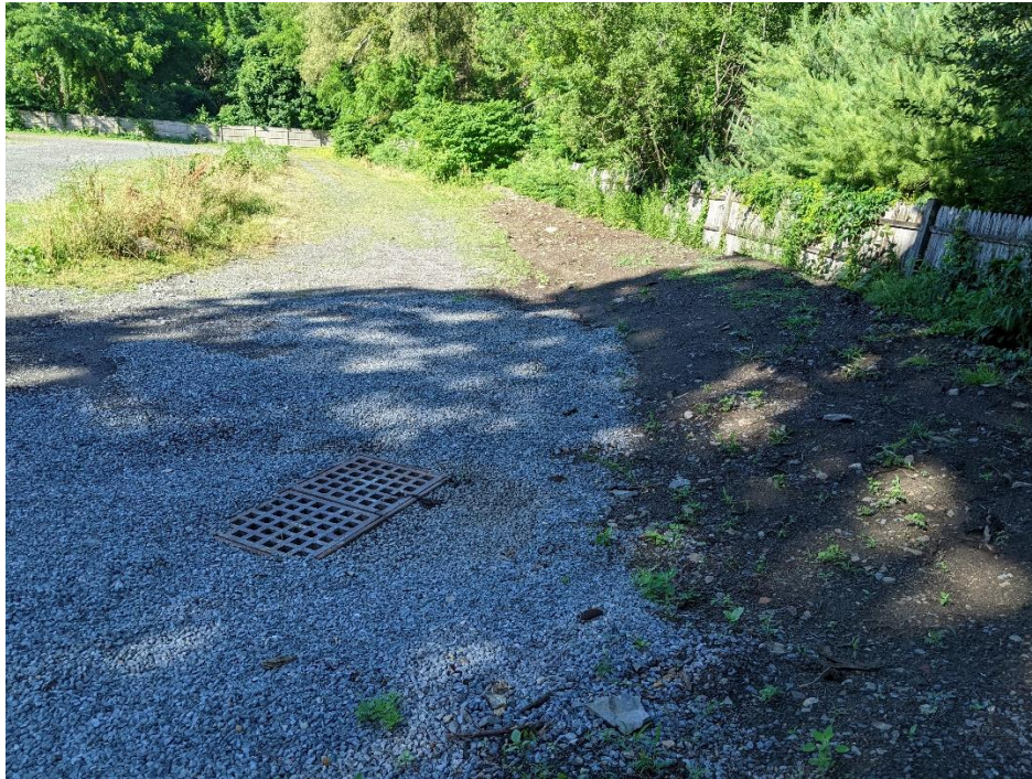
Existing double catch basin at the bottom of the sloped, gravel parking lot.
