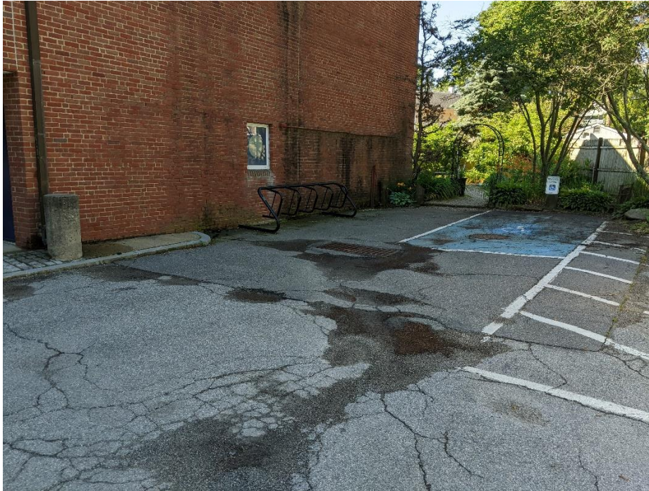
Water pools at the catch basins next to the library building. An elevated garden area at the far end of the lot could potentially be utilized for green infrastructure.
