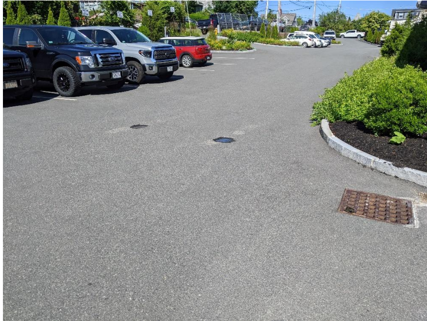
The parking area slopes down towards the harbor, with two catch basins on the paved section of the lot.
