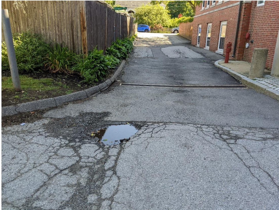
A long catch basin on the steep sloped driveway collects some runoff from the street. On the left, a vegetated island could be utilized for green infrastructure.
