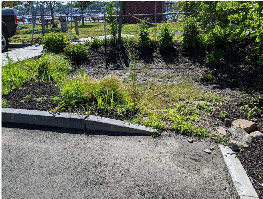
One of two bioretention areas that appears to not infiltrate due to signs of sediment setting on the pavement.
