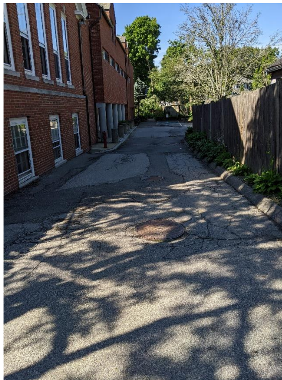
The building's gutter system discharges to the parking lot. Planter boxes could be placed along the edge of the building to collect and slow the discharge of roof runoff.
