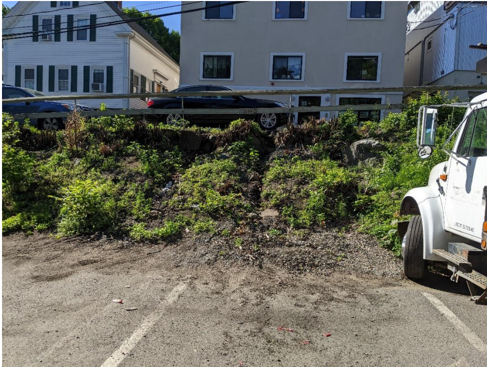
The steep slope along one edge is eroding.
