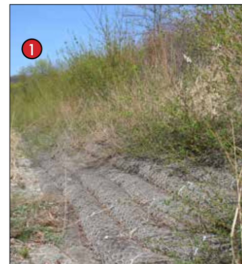
Fiber mats tucked into the embankment and planted to stabilize the slope.
