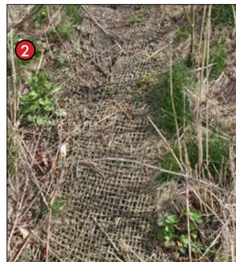
Patches of fiber are exposed due to erosion and lack of vegetation.
