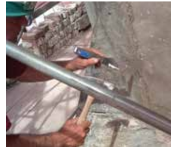
ABOVE: Meticulous care was taken in removing old mortar. Courtesy McGinley Kalsow & Associates
