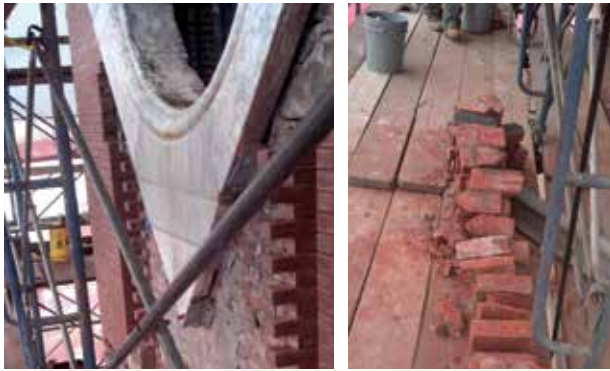
ABOVE LEFT: The outer wythe (layer) of brick removed at the marble “diamond” surrounding one of the clock faces. ABOVE RIGHT: Removed bricks were used as replacements whenever possible. Images courtesy McGinley Kalsow & Associates BELOW LEFT: Upon close inspection, the clock faces and dial markers showed signs of wear and tear. BOTTOM LEFT: All four clock faces (originally designed in upper and lower sections) were removed and restored by About Time Clock Restorations, Connecticut. The clock faces are made out of mahogany, with an applied crushed glass surface coating called “smalts.” New gold leaf was applied to the original bronze numerals and minute markers. Exact replicas of the clock hands were made from cypress and then gold leafed with smalts applied to the center sections. Both courtesy About Time Clock Restorations BELOW RIGHT: The restored clock faces and surrounding replica medallions. © Wednesdays in Marblehead
