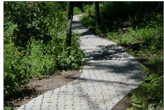
New buildings with quasi-public open space, top. Permeable pavers reduce stormwater runoff.
